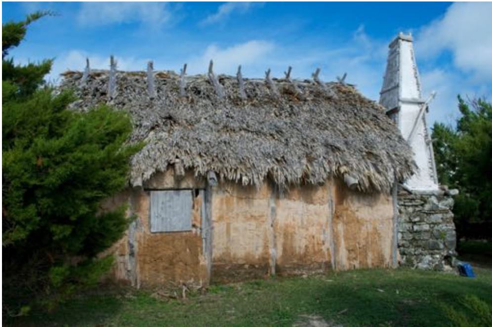
Figure 20 Replica wattle and daub house thatched with palmetto leaves. At Carter House Museum. Photo by Saskia Wolsak.
